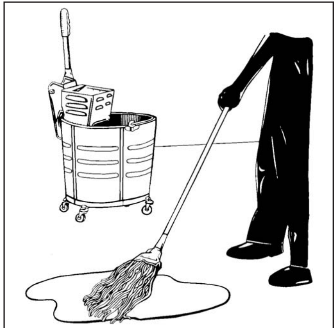
Figure 4. Applying floor finish.
